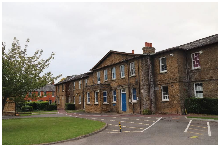
Administration Block, St Mark's Hospital
