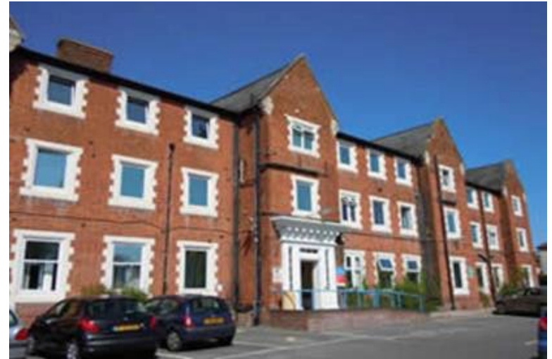
Main block frontage, Wokingham Community Hospital
