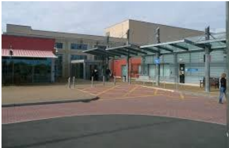
Frontage of West Berkshire Community Hospital
